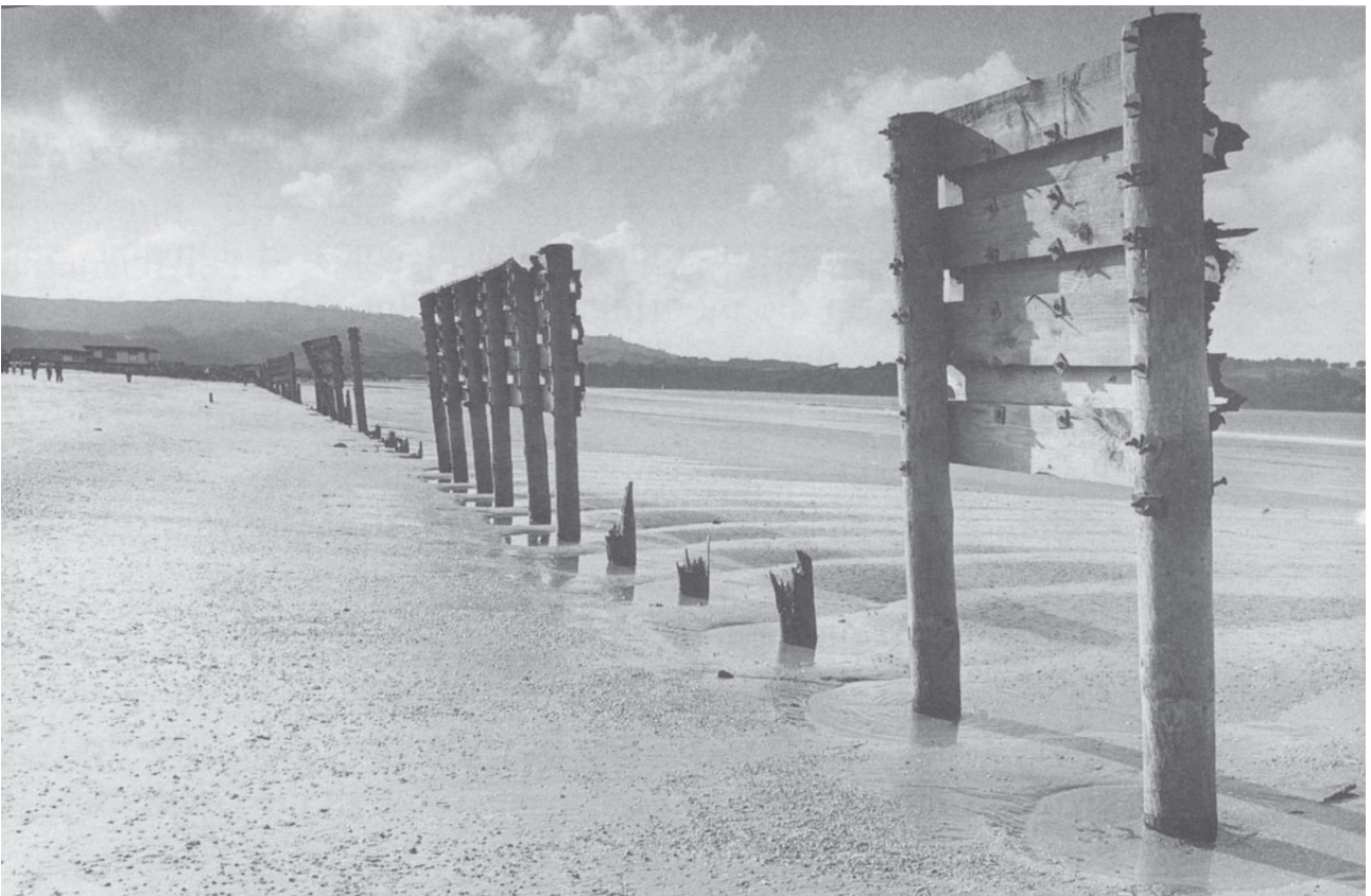
(Below): The July 1978 storm demolished the wall and removed more sand from the beach. Photo courtesy of Cliff Grant.
